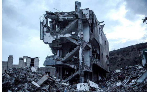
Residential building destroyed by an airstrike by the Saudi Arabia/UAE-led coalition on 25 August 2017 on Faj Attan, Sana'a, Yemen, killing 16 civilians and injuring 17 more. © Rawan Shaif
